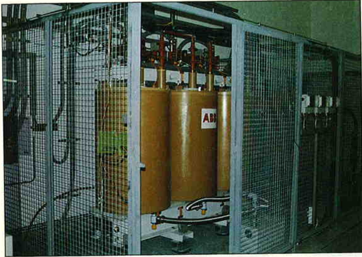
[4] The 630-kVA demonstration transformer based on high-temperature superconductor windings is presently under test by ABB, ASEA Brown Boveri Ltd., on the grid in Geneva, Switzerland. Designed to convert power from 18.7 kV to 420 V, its superconducting windings are made of power-in-tube BSCCO-2223.
