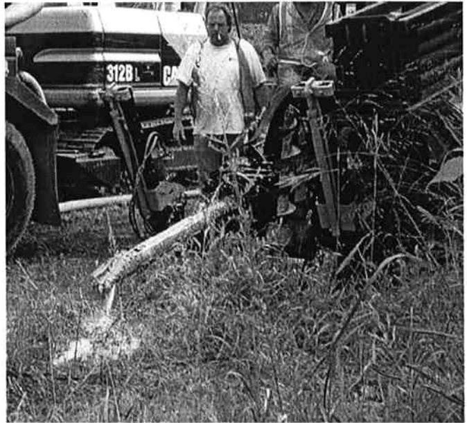
Fig. 3. Horizontal directional drilling of the conduit path parallel to the railroad.
