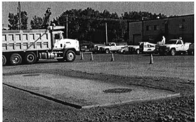
Fig. 4. Installed underground vault waiting for blacktopping.
