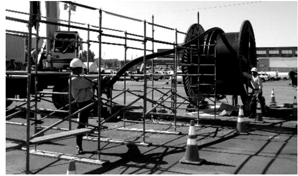
Fig. 2. 30-meter YBCO Cable installation
