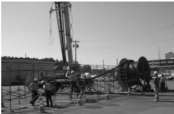
Fig. 15. Installation of the 30 m long cable made by Sumitomo Electric with nearly 10,000 m of SuperPower's 2G HTS wire.
